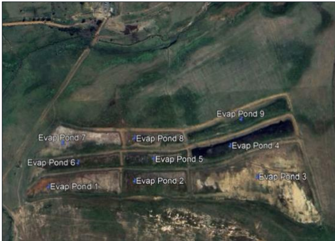
Figure 2-13 – Existing evaporation dam indicating the nine compartments (evap pond 1-9 are the nine compartments of the existing evaporation dam).
