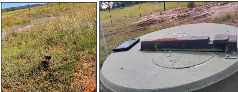
Figure 2-6 – Photo of borehole BHR4 (left) and borehole BHR4 installed with a pump (right)
