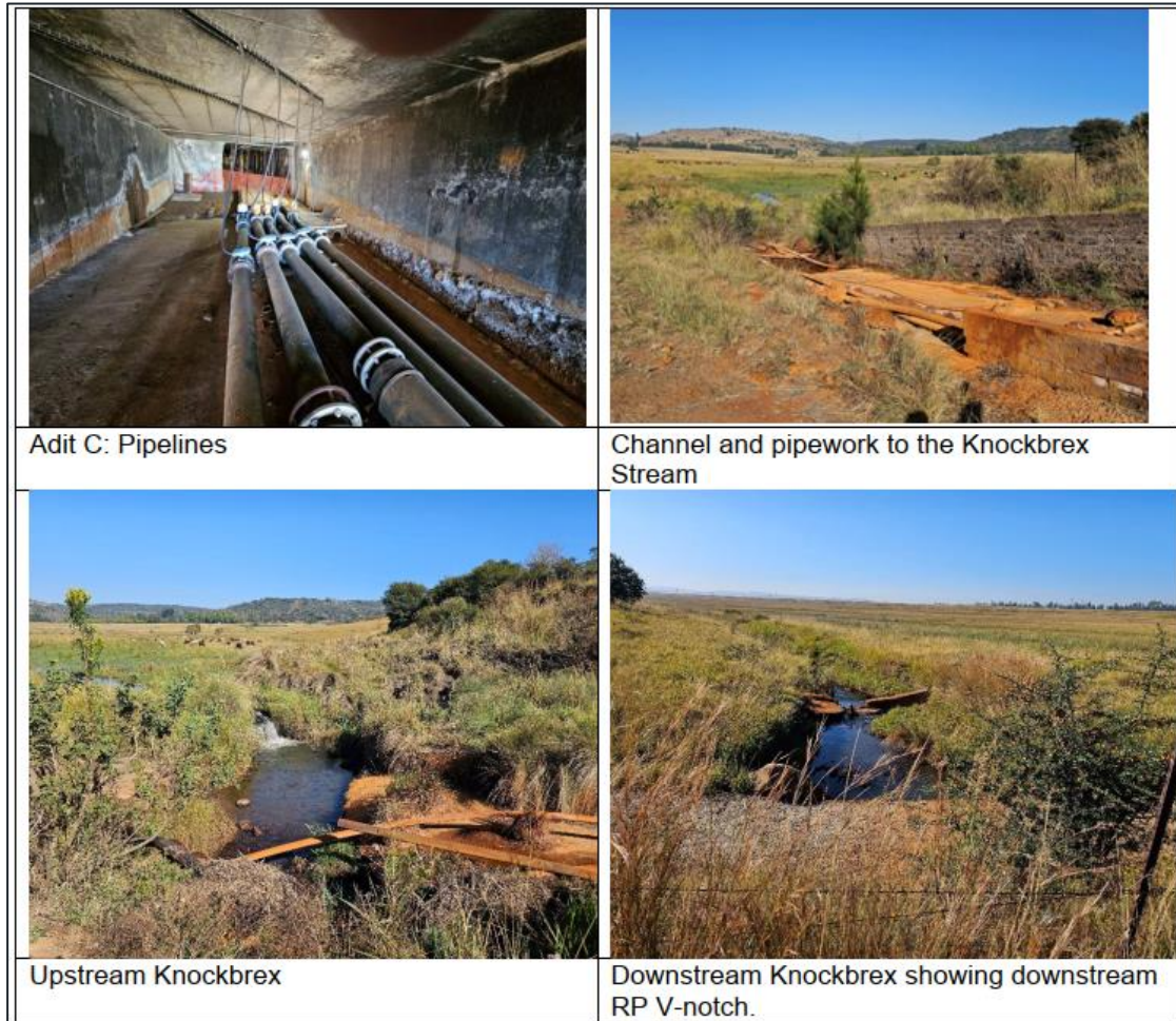
Figure 2-4 – Controlled discharge from the main Adit to the Knockbrex, 2023
