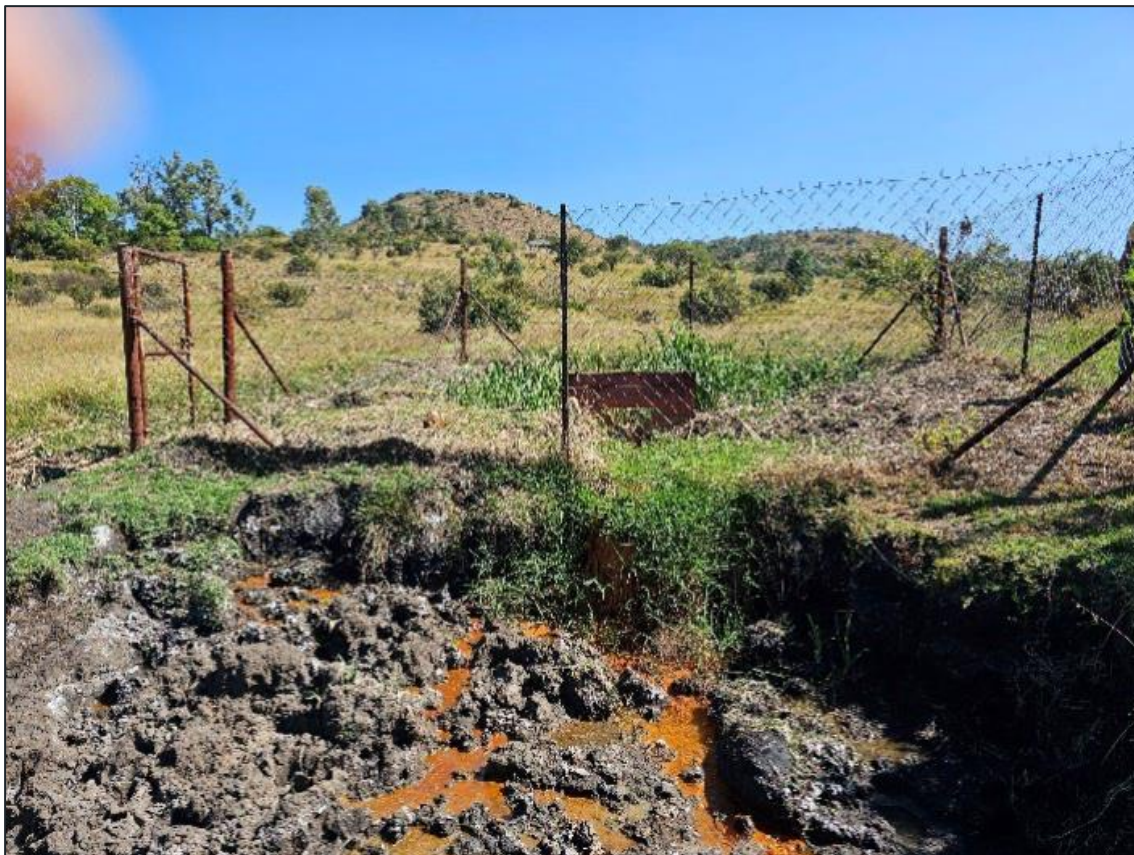
Figure 2-7 – Harris Adit, April 2023
